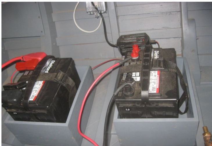
Photo 10 New batteries and connection to generator.
